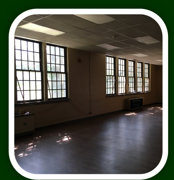
The new boys' dormitory floor with LVT flooring!
